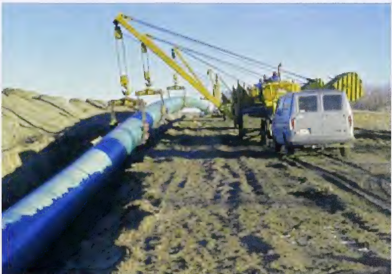
Photo 16 Lowering in large diameter pipe.
